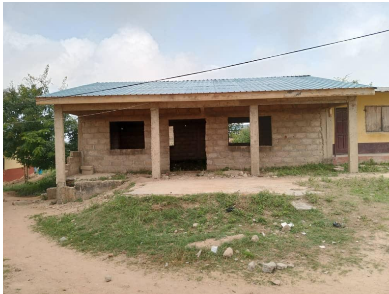
What the building looks like, with a roof over it.
