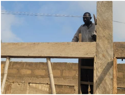
Carpenter at work standing on a raised platform.
